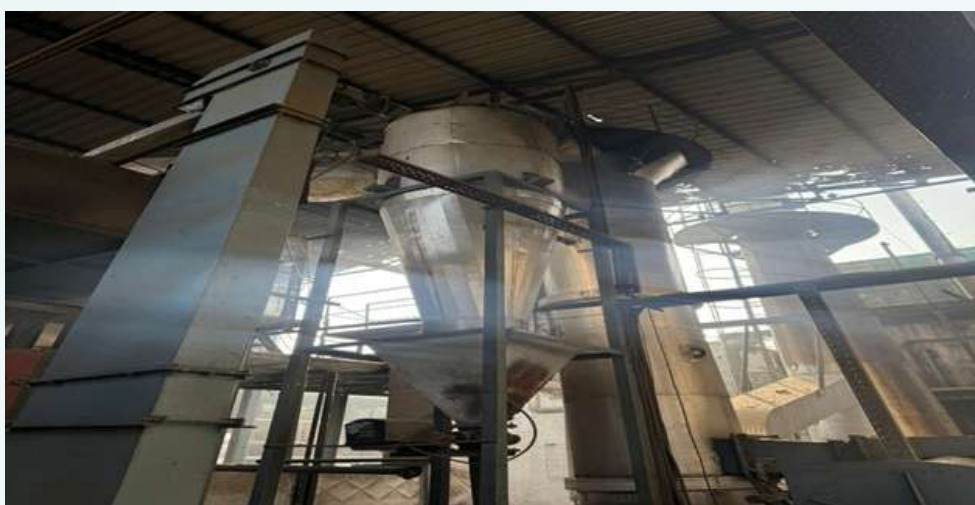
Cyclone Centrifugal installed at boiler to trap solid particle to approach Chimney
