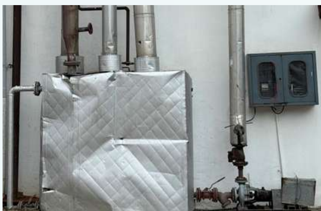
Condensate Storage tank and Pump System
